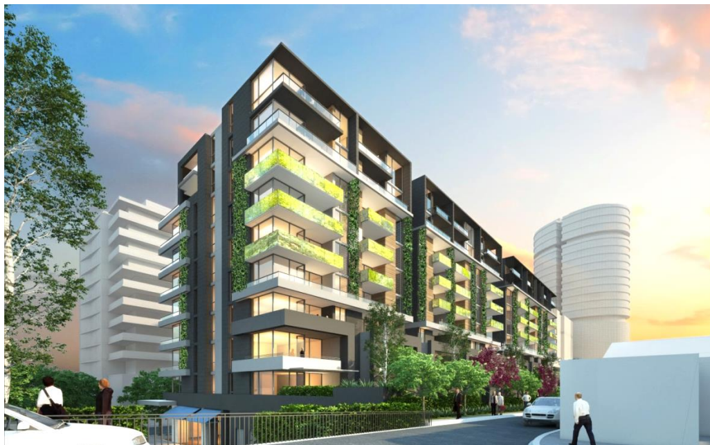
Figure 24: Portman Lane Elevation of Buildings 16A and 16B to the south-east, subject to conditions in the process of being satisfied for the podium wall and laneway landscaping.
